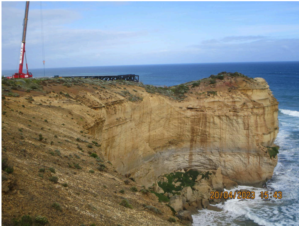
20-4-2023 – the base of the viewing platform is in place adjoining cliff collapses on both sides. Photo PCCG Inc
